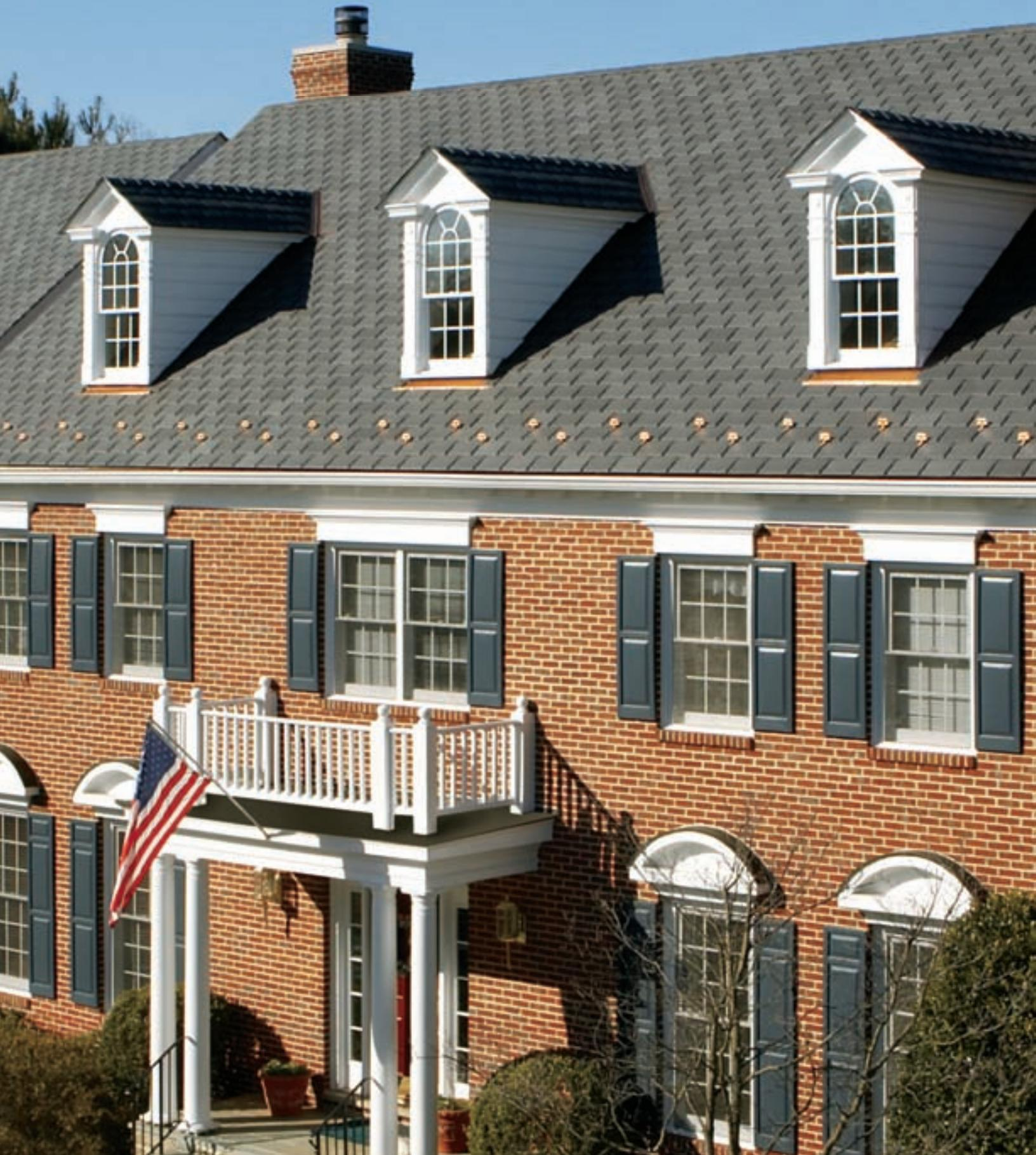
Symphony adds authenticity with standard 12" slate widths or multiple-width bundles of 6", 9" and 12" widths and color blends that allow multiple installation options, including graduated and random patterns.
